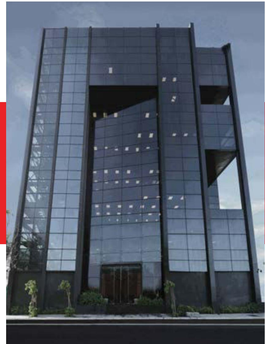
Being one of the tallest buildings in the area, without any surrounding walls and with a high window-to-wall ratio, keeping the heat levels low was a daunting task; we had a significant success by using double glazed windows, with a thin layer of argon in between; however, the stifling Sri Lankan sun still forces the air conditioning to account for more than 70% of the building's energy requirement.
